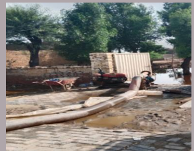
Dewatering activity ongoing at GD Jaffereabad
